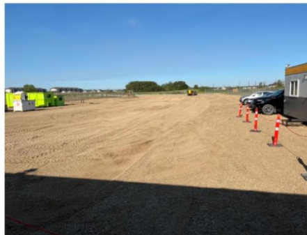
Site Parking and Laydown Area Photo July 27, 2023
