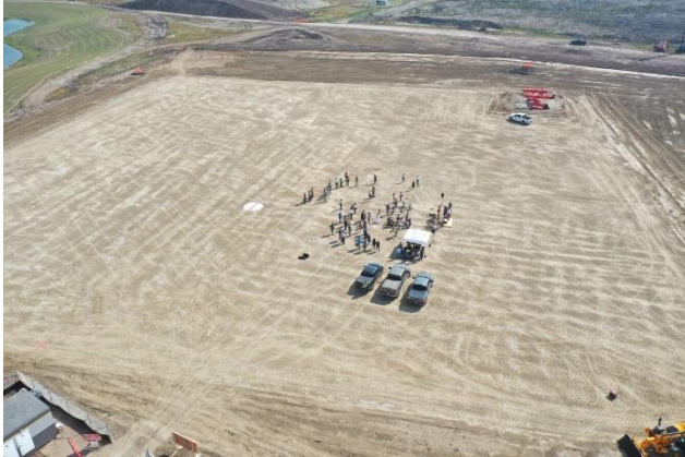
Drone footage of Groundbreaking Ceremony August 29, 2023
