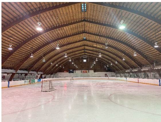
Figure 28: Interior View of Roof
