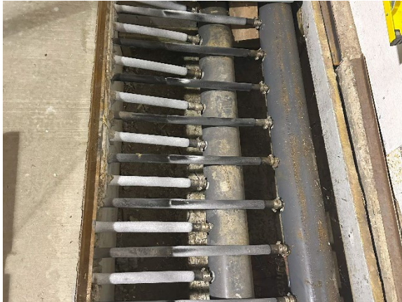
Figure 49: Header Trench within Apron Slab
