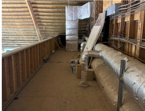
Figure 50: Mezzanine (Inaccessible), Above Lobby
