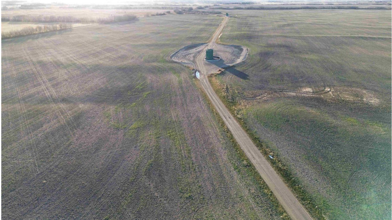
Photograph 23: Looking southwest towards Oil and Gas installation within 1 & 2-22-49-01 W4M
