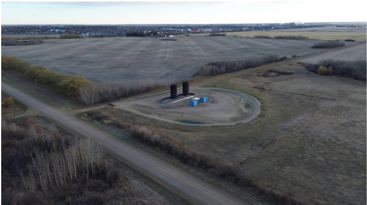
Photograph 10: Looking northeast towards Oil and Gas installation within 5-24-49-01 W4M
