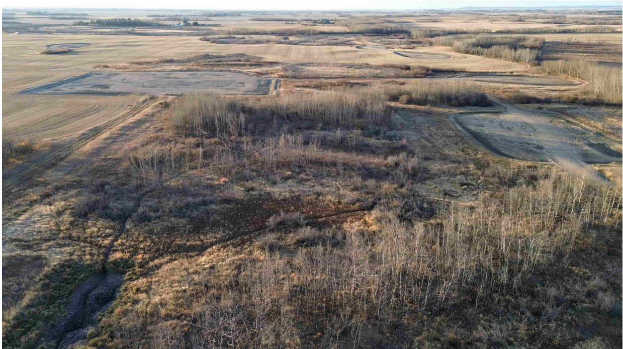
Photograph 30: Looking south towards Oil and Gas installation within 2 & 7-34-49-01 W4M
