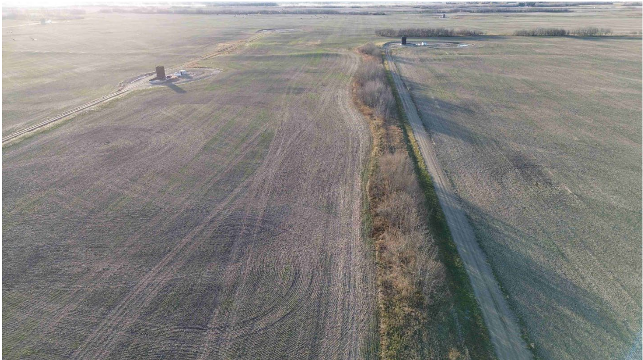
Photograph 22: Looking west towards Oil and Gas installation within NE & SE-22-49-01 W4M
