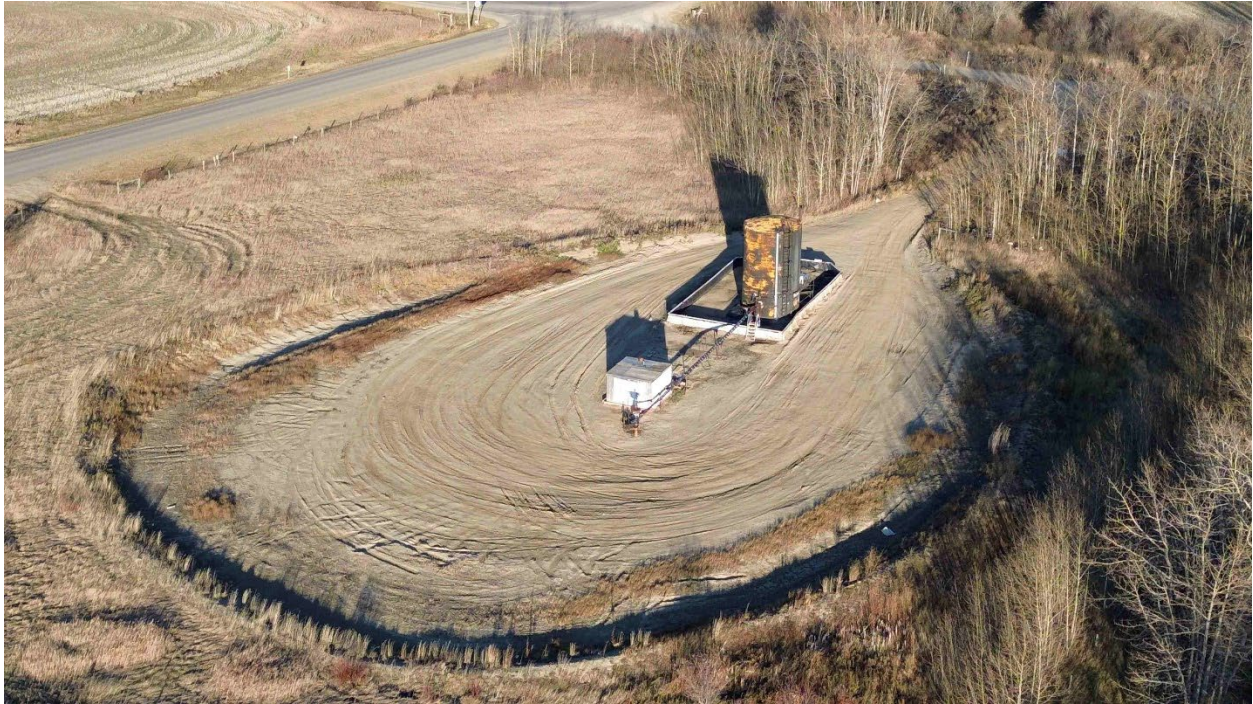
Photograph 21: Looking northeast towards Oil and Gas installation within 16-22-49-01 W4M
