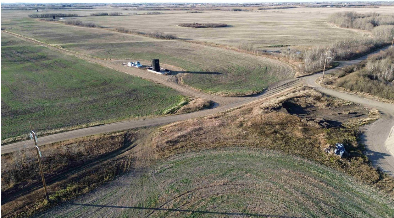
Photograph 4: Looking northwest towards Oil and Gas installation within 8-22-49-01 W4M
