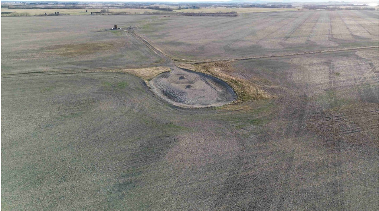
Photograph 5: Looking southwest towards Oil and Gas installation within 2-23-49-01 W4M
