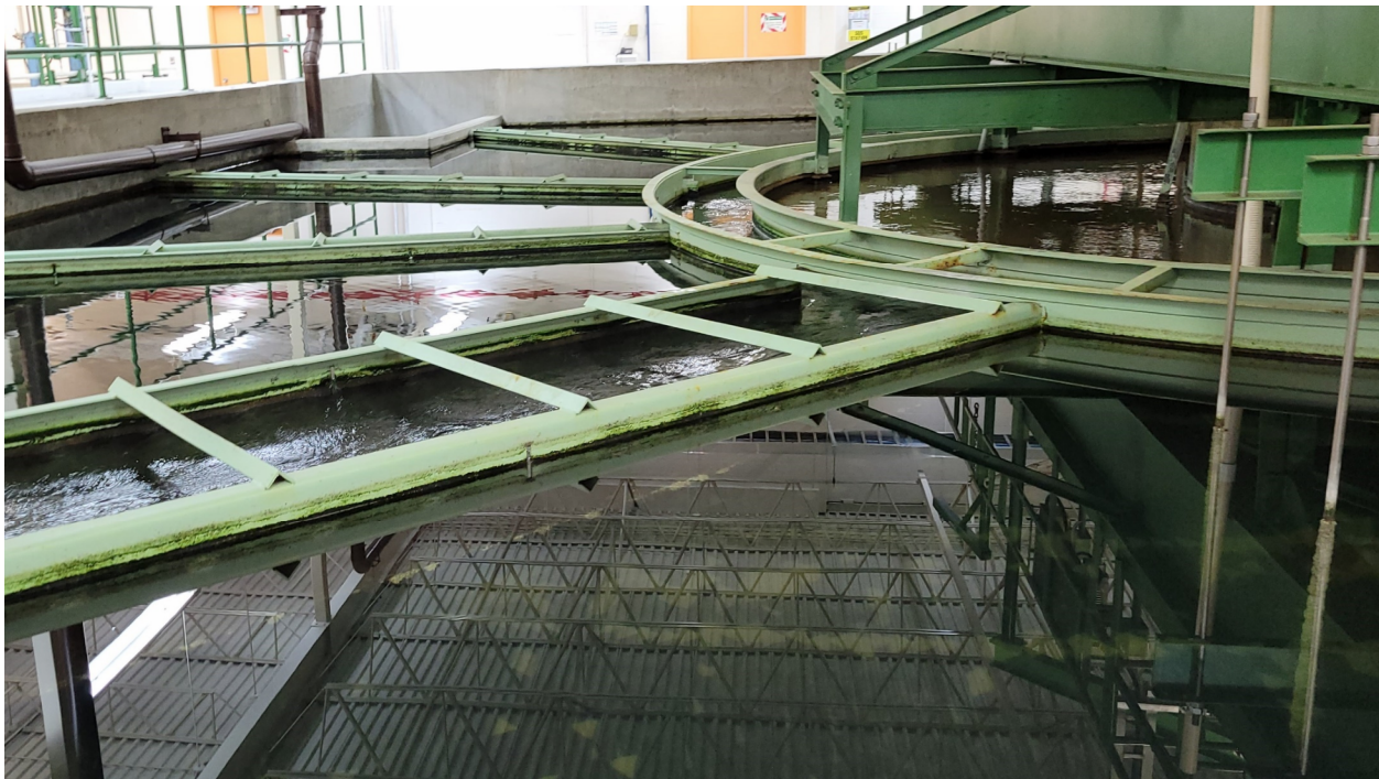
Figure 4.4 Solids Contact Clarifier
