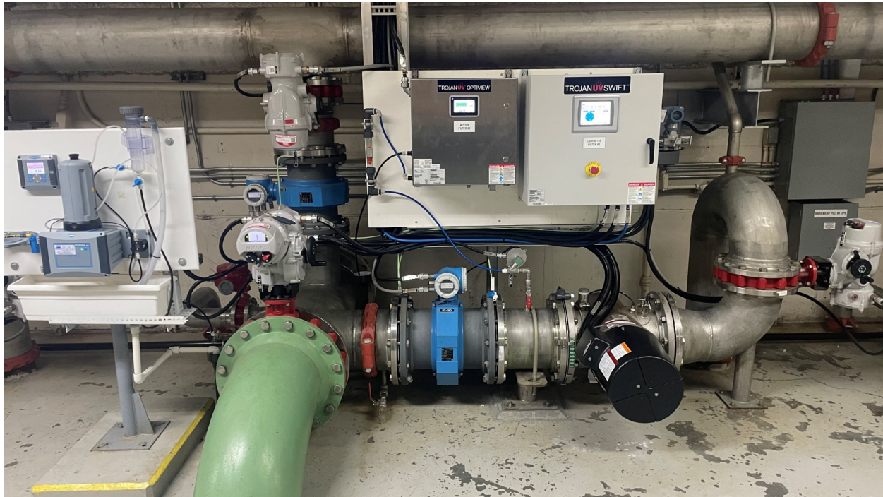
Figure 2.5 UV Reactor & Filter Outlet Pipework
