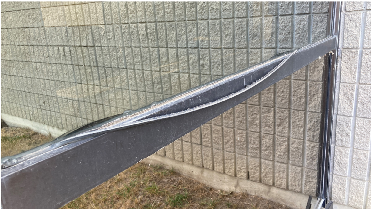
Figure 4.9 Curtain Wall Damage
