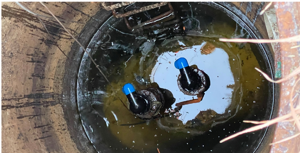
Figure 4.2 Flooded Raw Water Pipeline Vault
