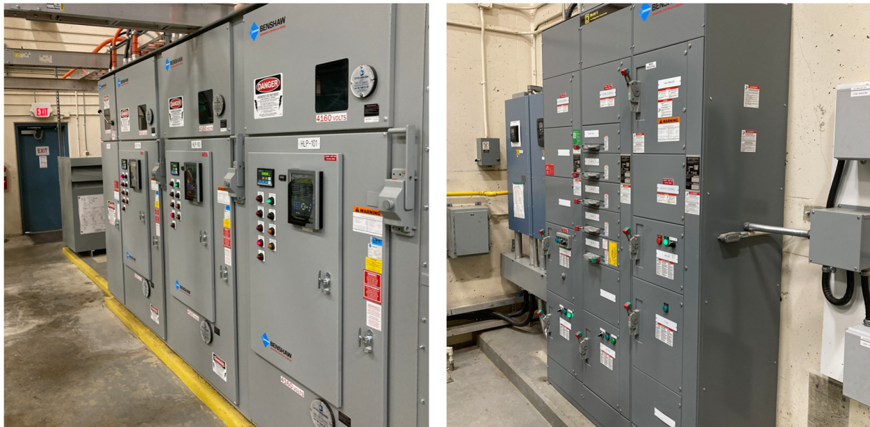
Figure 4.10 River Pumphouse 4160v Switchgear and 600v Motor Control Centre
