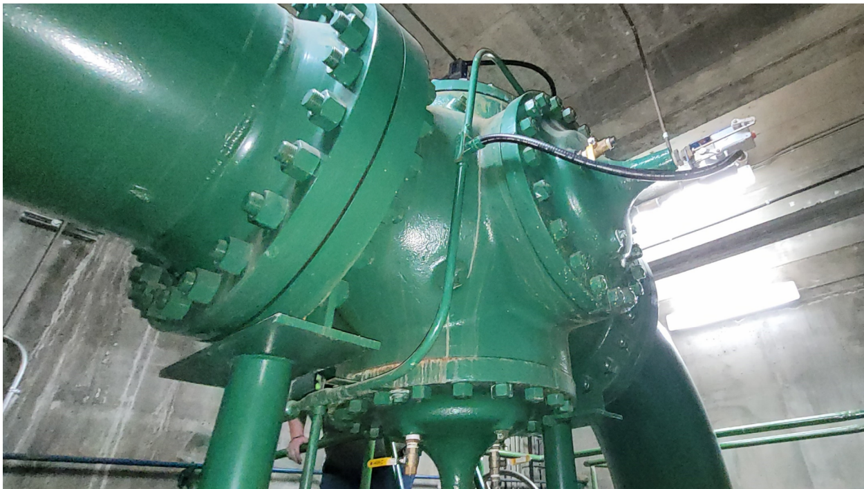
Figure 4.3 Vault 5 Hydraulic / Pressure Control Valve
